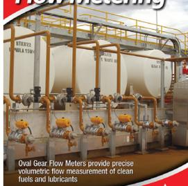
Oval Gear Flow Meters provide precise volumetric flow measurement of clean fuels and lubricants
